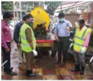
Sanitation work in progress
